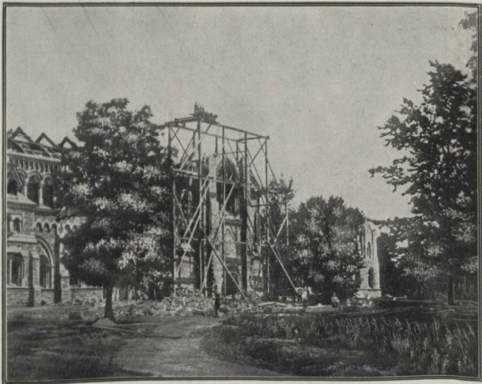
THE MAIN TOWER IN COURSE OF ERECTION—THIS PHOTOGRAPH SHOWS THE TREES WHICH WERE CAREFULLY LEFT IN POSITION AND PRESERVED TO ADD TO THE APPEARANCE OF THE BUILDING. ALL THESE HAVE SINCE BEEN REMOVED
