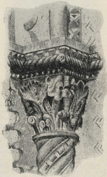
CAPITAL FROM MAIN ENTRANCE, SHOWING FOLIAGE CARVING WITH GEOMETRICAL FORMS ON COLUMN AND ABACUS
