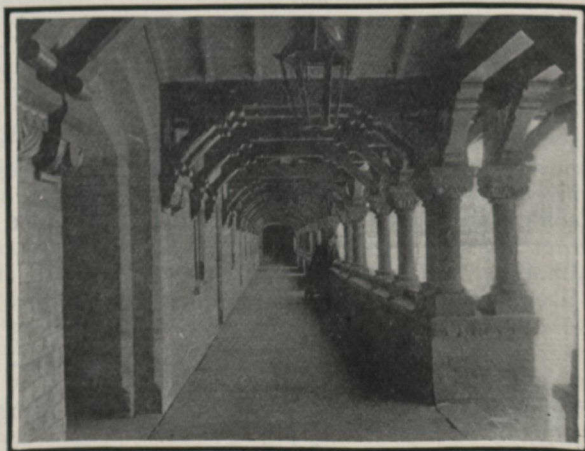
CORRIDOR OVERLOOKING INTERIOR QUADRANGLE, BUILT IN WOOD
