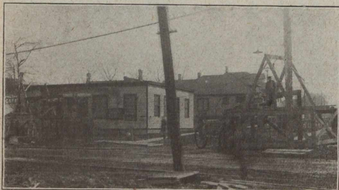
HOIST FOR HANDLING EXCAVATED MATERIAL
