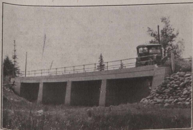
Fig. 5.—Concrete Beam Bridge in Cumberland County.
