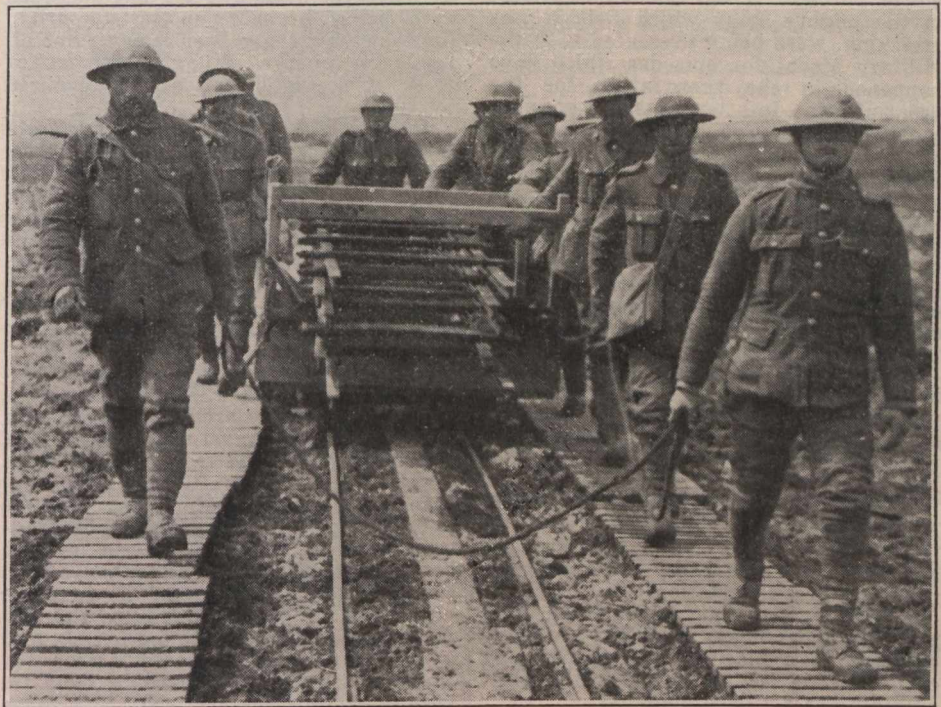
Light railway laid over captured ground on the British Western Front Official photograph issued on behalf of The Press Bureau. Crown copyright reserved. Loaned by C.P.R.
