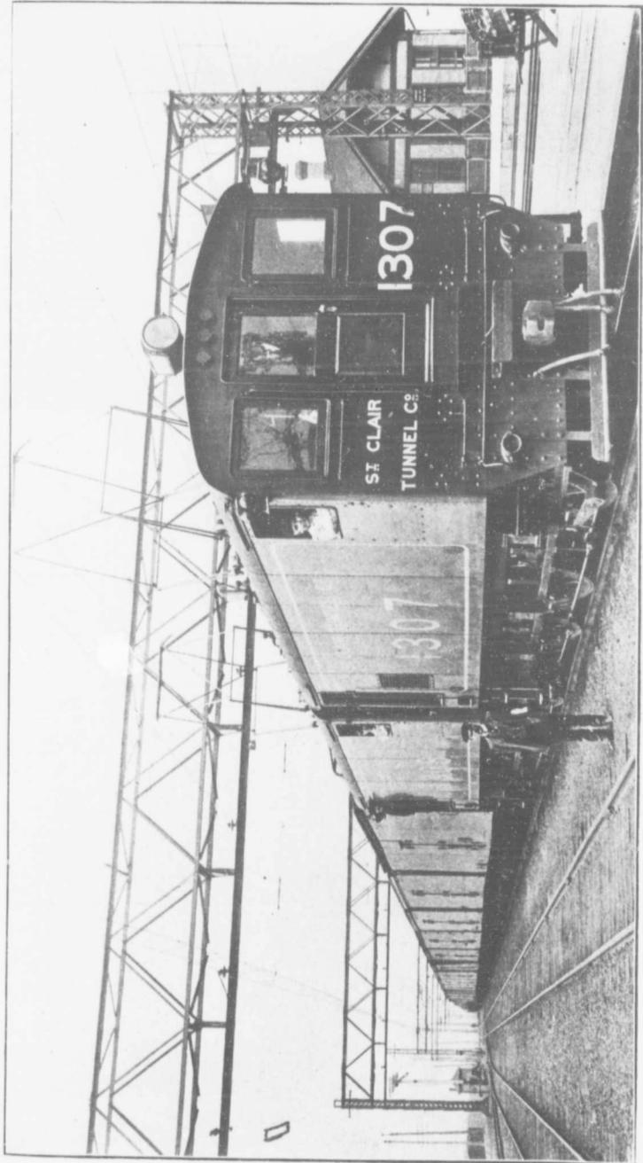
Grand Trunk freight train with electric locomotives for operation of trains through St. Clair Tunnel. Photograph taken at Sarnia Tunnel Station.
