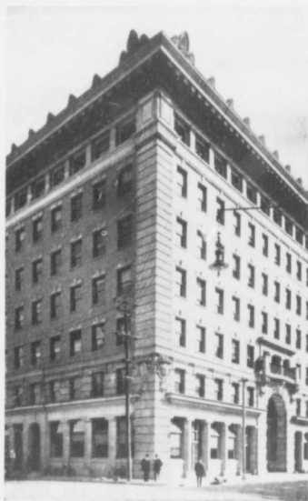
GRAIN EXCHANGE BUILDING
