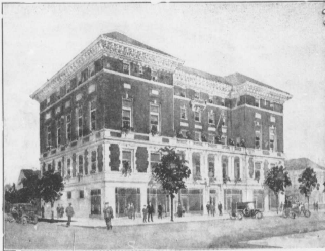
Handsome building to be erected by The Columbus Hall Association, Ltd., of Winnipeg, John D. Athinsson & Company Architects.
