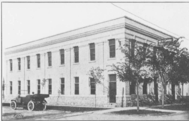
WEST CANADA BUILDING
