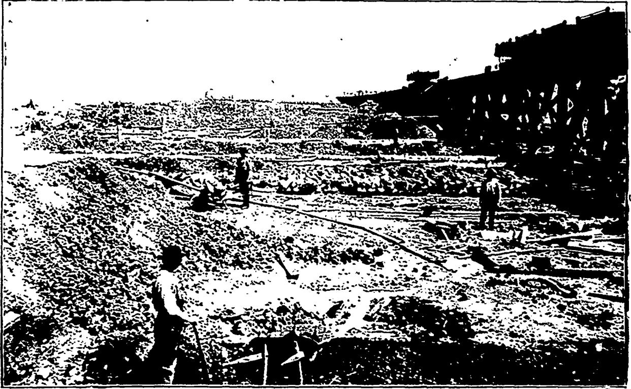
Canadian Copper Co.—Roasting Nickel Ore at Copper Cliff, Sudbury, Ont.
