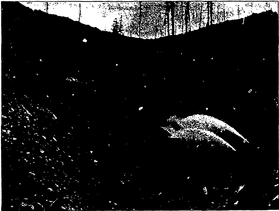
Cariboo Hydraulic Mine. Giants discharging 2000 miners inches of water in No. 1 Pit. August, 1896.
