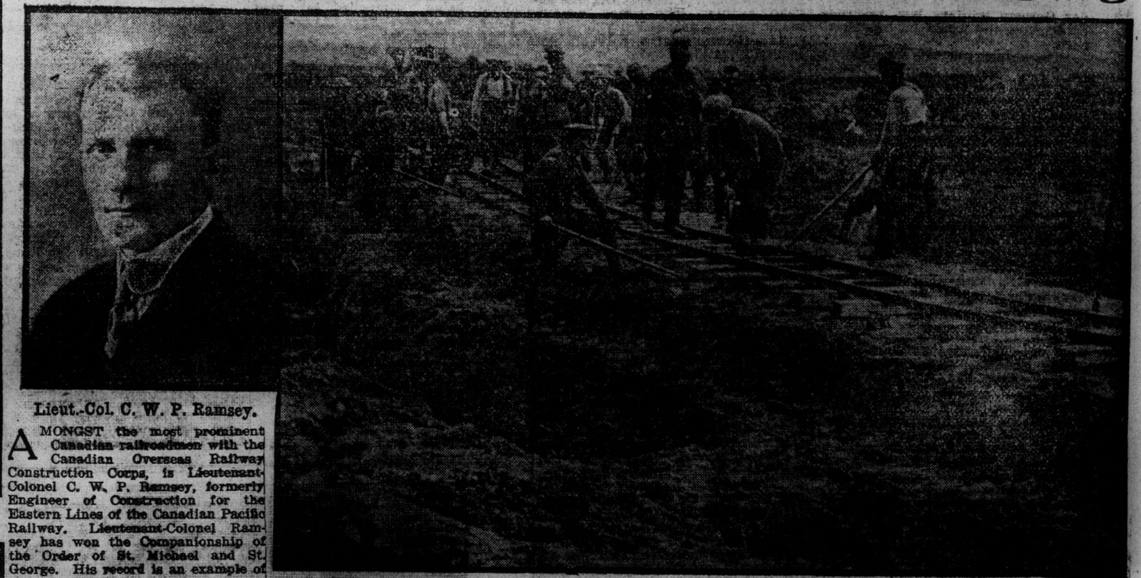
The Railway Construction Corps lays the rails as fast as the armies advance. —Photo by courtesy of C. P. R.
