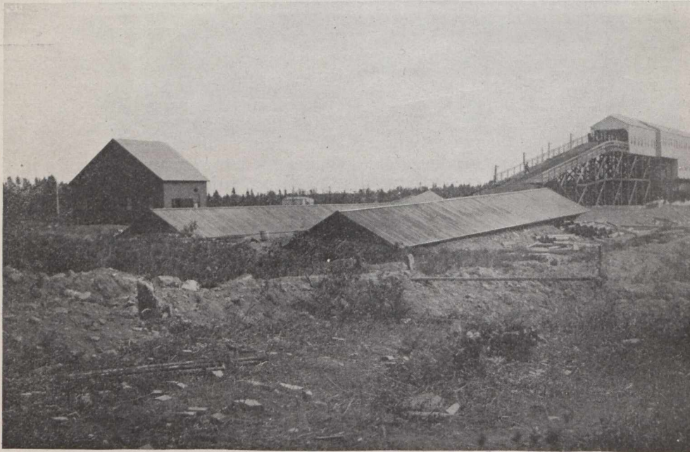
Mouths of Slopes, Compressor House and Bankhead—Dominion No. 21 Colliery.
