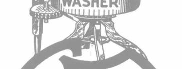
The New Century Washers solves the washing problem. It eliminates slavish, arduous toil and reduces manual labor to the minimum. The city water pressure furnishes the power that is transmitted by the New Century water motor.
