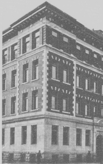
CORNER OF McDERMOT AVENUE AND CHARLOTTE STREET
