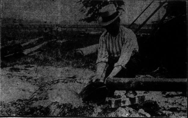
No. 6 well at the Rockwood Oil Company's property at Glencoe, showing oil and will be further sunk to the 375-foot level.
