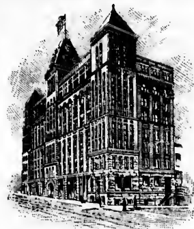
MARQUAM GRAND OPERA HOUSE.
