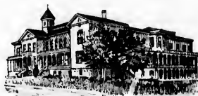
GOOD SAMARITAN HOSPITAL, PORTLAND.
