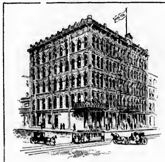
THE HOLTON HOUSE, PORTLAND.
