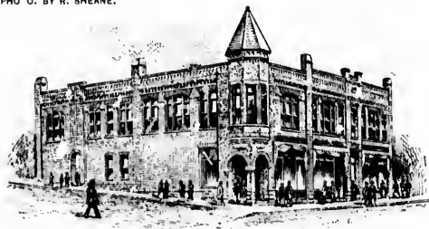
CHEHALIS IMPROVEMENT CO.'S BUILDING, CHEHALIS.
