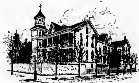
ST. VINCENT'S HOSPITAL, PORTLAND.
