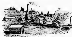
DRY CRUSHING CHLORIDIZING MILL, BI-METALLIC MINING CO., PHILLIPSBURG.
