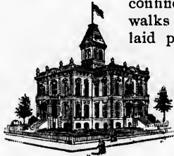
YAMHILL COUNTY COURT HOUSE, McMINNVILLE
