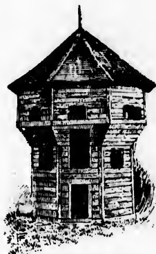
OLD BLOCK HOUSE, NANAIMO.
