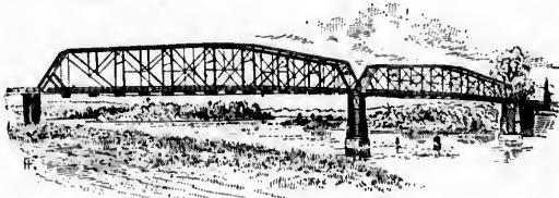
BRIDGE ACROSS WILLAMETTE RIVER, SALEM.
