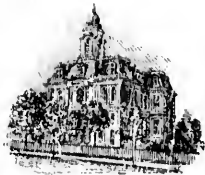
COURT HOUSE, SALEM.
