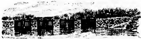
UPPER VIEW, MAIN HEADGATE, GREAT WESTERN CANAL, IDAHO FALLS.
