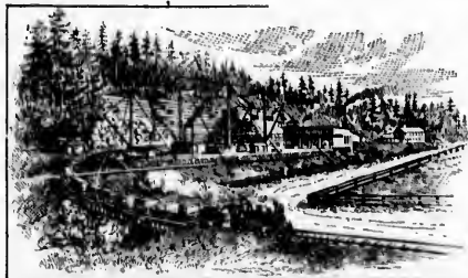
EUREKA SANDSTONE CO.'S WORKS, TENINO.
