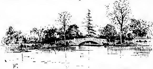
BRIDGE AT BEACON HILL PARK, VICTORIA.
