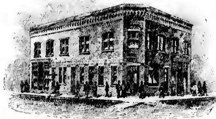
BIG BEND NATIONAL BANK BUILDING, DAVENPORT.
