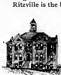
SCHOOL HOUSE, RITZVILLE.
