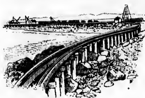
WORKING ON JETTY-MOUTH COLUMBIA RIVER.
