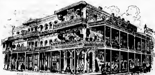
BUILDING OCCUPIED BY CHINESE, PORTLAND.
