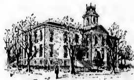
PARK SCHOOL, PORTLAND.
