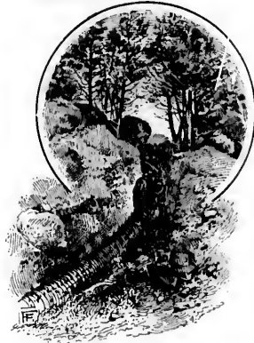
24-INCH REDWOOD MAIN FROM RESERVOIR TO CITY WATER WORKS, BUTTE.
