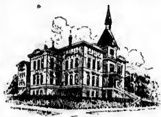
FAILING SCHOOL, PORTLAND.
