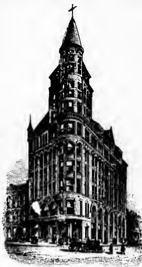
REVIEW BUILDING, SPOKANE.
