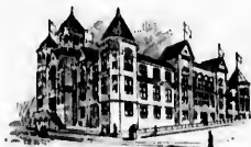
EXPOSITION BUILDING, TACOMA.
