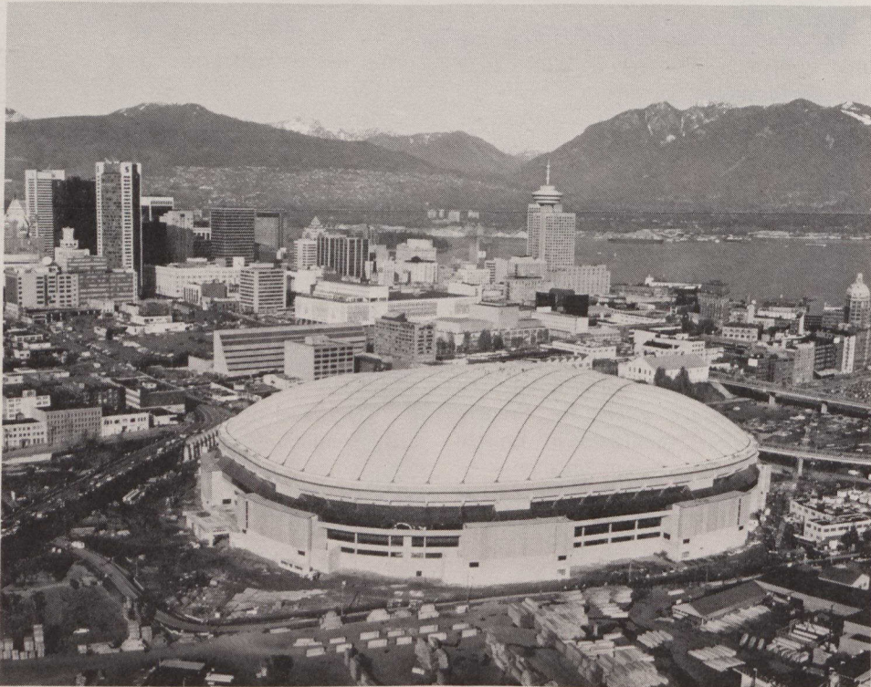
Roof covers 60 000-seat stadium over ten acres and weighs 123 tonnes.
