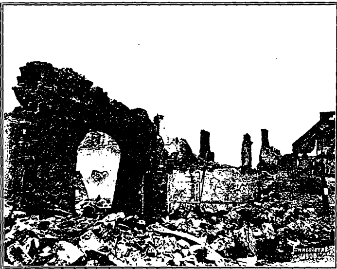
PARTIAL VIEW OF WINDSOR HOTEL SHOWING THE HAVOC WROUGHT BY THE FLAMES UPON AN EXCEPTIONALLY HEAVY PIECE OF CORNICE-STONE MASONRY. PHOTO BY P. F. PINSONNEAULT.
