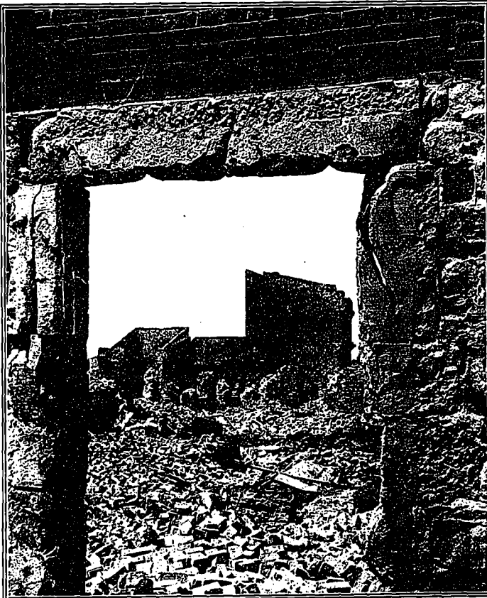
DOOR OF MARKET PLACE IN WHICH IS FURTHER SEEN THE EFFECT OF THE FIRE ON THE HEAVY STONE MASONRY. PHOTO BY P. F. PINSONNEAULT.
