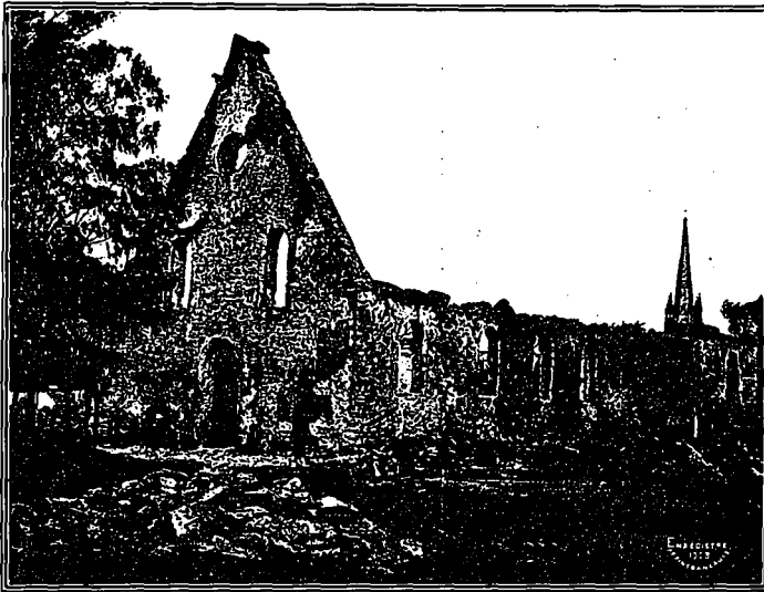
THE RUINS OF THE HISTORIC PARISH CHURCH WHICH OWES ITS DESTRUCTION TO THE FIRE FINDING ITS WAY INTO THE INTERIOR THROUGH THE BELFRY AND UNPROTECTED DOOR, AND WINDOW OPENING. IT WAS KNOWN AS THE SECOND OLDEST CHURCH IN CANADA. PHOTO BY P. F. PINSONNEAULT.
