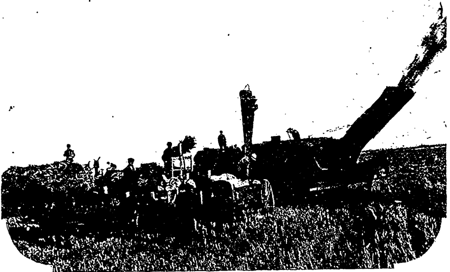
Showing the high-bagger, an automatic device which elevates the grain, weighs a bushel at a time, and drops it down the chute into a bag held by a man in the waggon.
