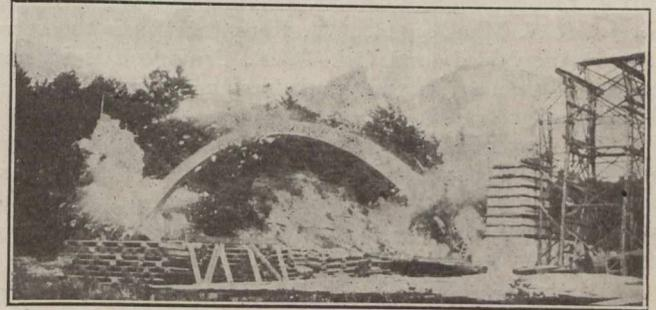
Readers are referred to the article. The illustration herewith is descriptive of the method of dynamiting and shows the position and simultaneous explosion by electric spark of the shots placed in the crown and near the haunches of the arch.
