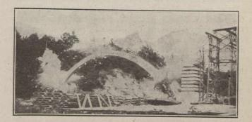
Readers are referred to the article. The illustration herewith is descriptive of the method of dynamiting and shows the position and simultaneous explosion by electric spark of the shots placed in the crown and near the haunches of the arch.
