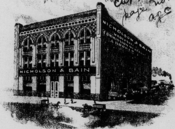
Bannatyne St., East, Transfer Track
