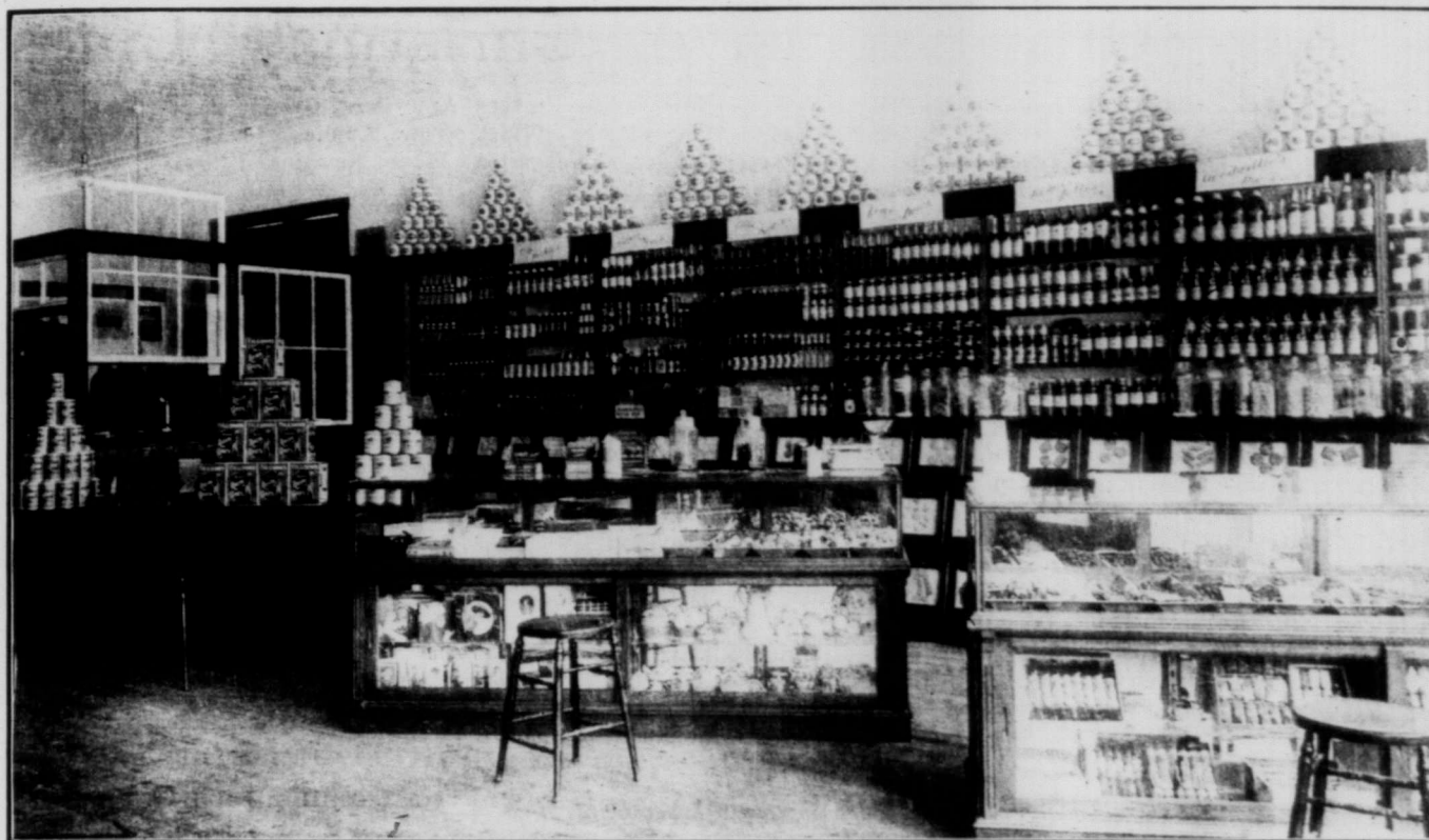
An interior view of Cain Bros. new store in Yarmouth, N.S., showing bin fixtures, silent salesman and metal ceiling.
