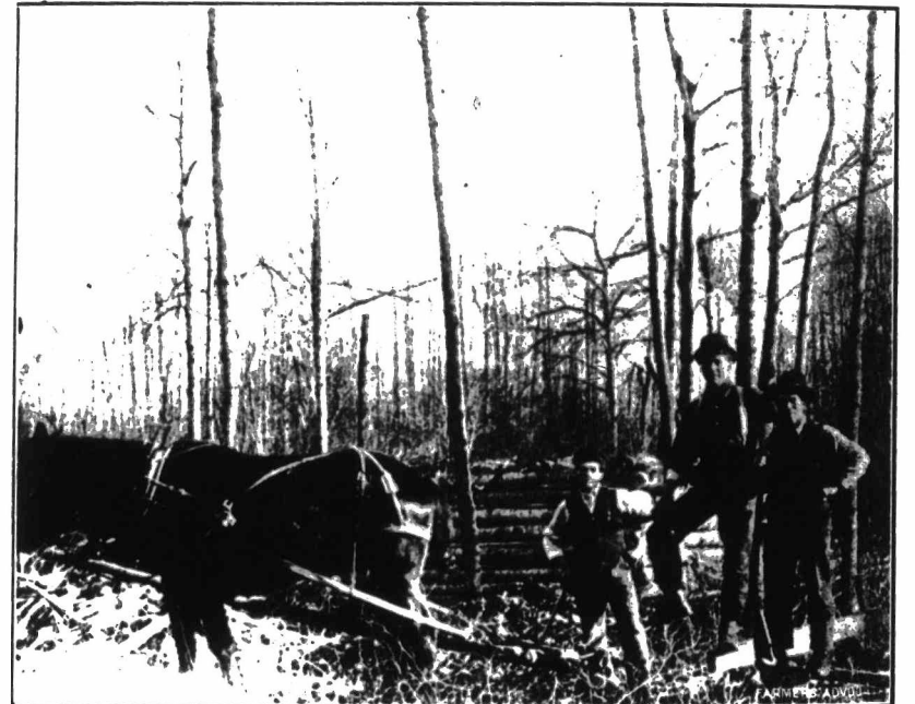
CLEARING THE ROAD AND PREPARING FOR CORDUROY IN ROSEDALE MUNICIPALITY
