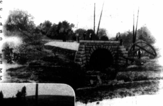
Two G. T. Ry. Culverts near Newtonville, Ont. 8 and 20 foot openings
