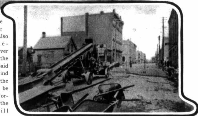
Showing Mixer and Concrete Placer at Work
