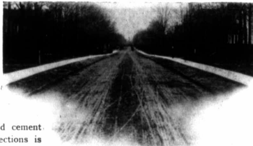
Grange Street, Stratford Ont. Guelph Pavement Co.
