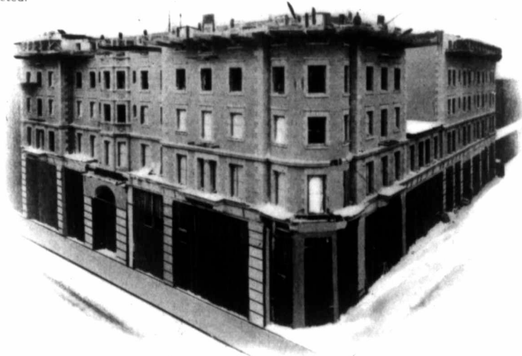
King Edward Hotel, Toronto, Ont. Hilsley & Horne, Ltd., General Contractors
