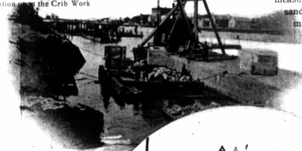
Ten Ton Concrete Blocks holding Crib in position for filling
