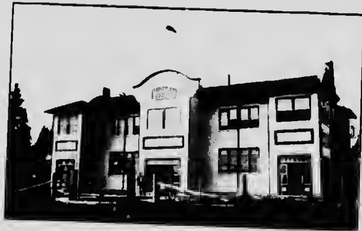
Agricultural Hall, Coquitlam, B. C.
