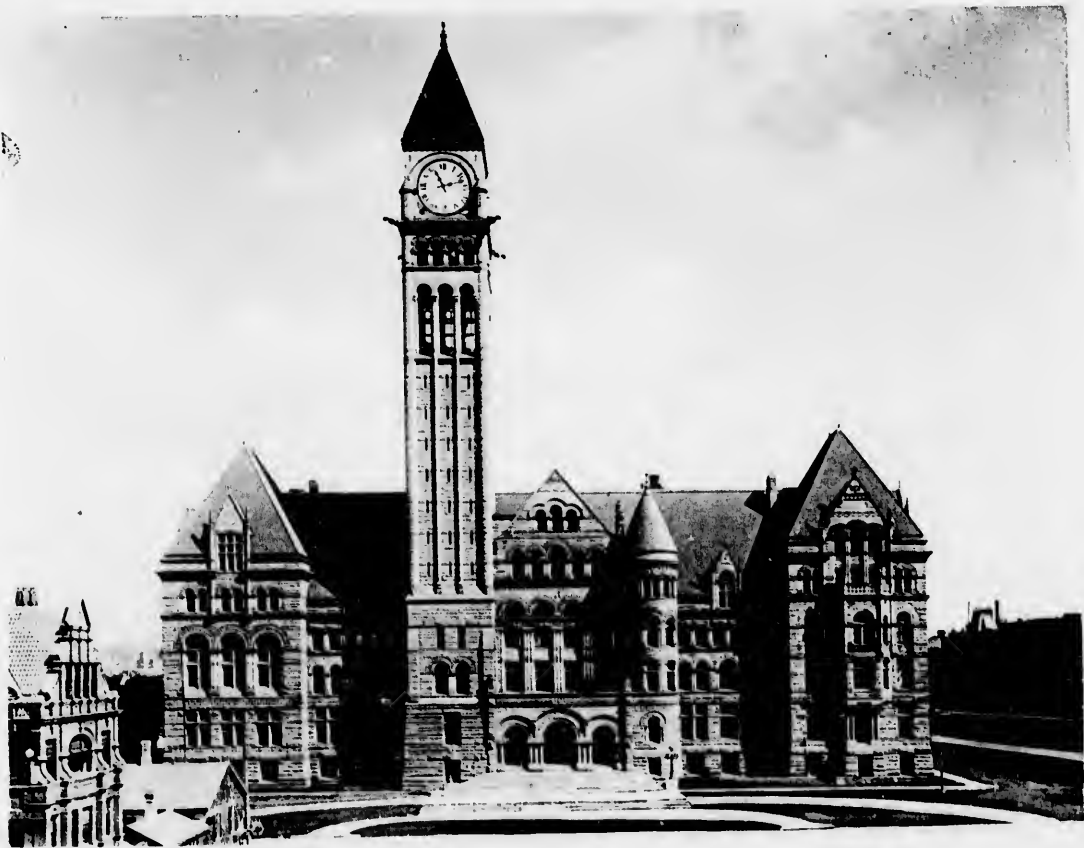
NEW MUNICIPAL AND COUNTY BUILDINGS
