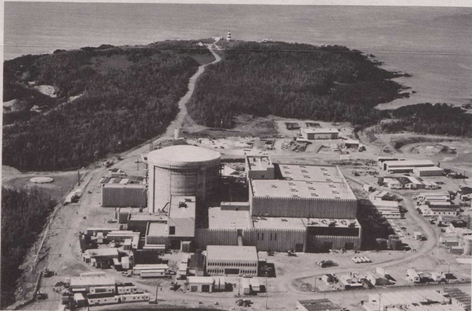
Point Lepreau, Quebec, a 600-megawatt Candu nuclear generating station.
