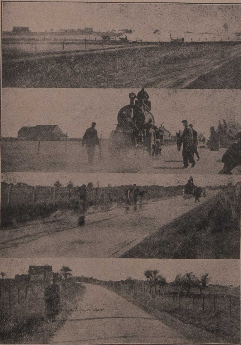
5.—Road Edward VII.—Parish of Napierville (Napierville). Road treated with fluxphalte (from top to bottom) (a) Sweeping of the road made with the mechanic sweeper; (b) application of fluxphalte by means of a pressure distributor; (c) application of gravel on fluxphalte; (d) completed road.
