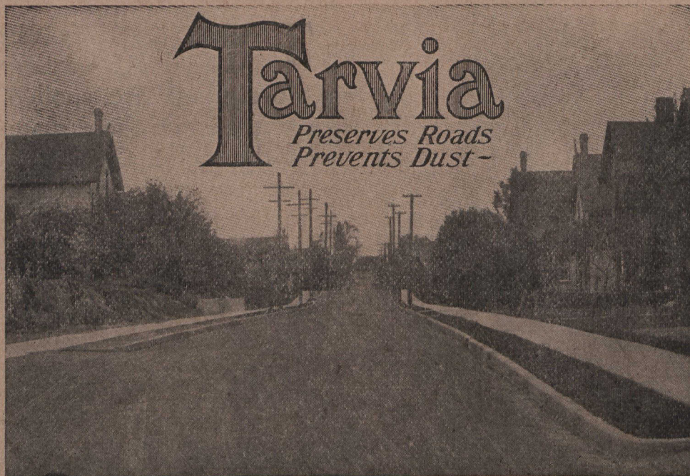
Strange St., Berlin, Ontario. Constructed 1915 3 inch Tarvia Penetration Top on 5 inch concrete base.
