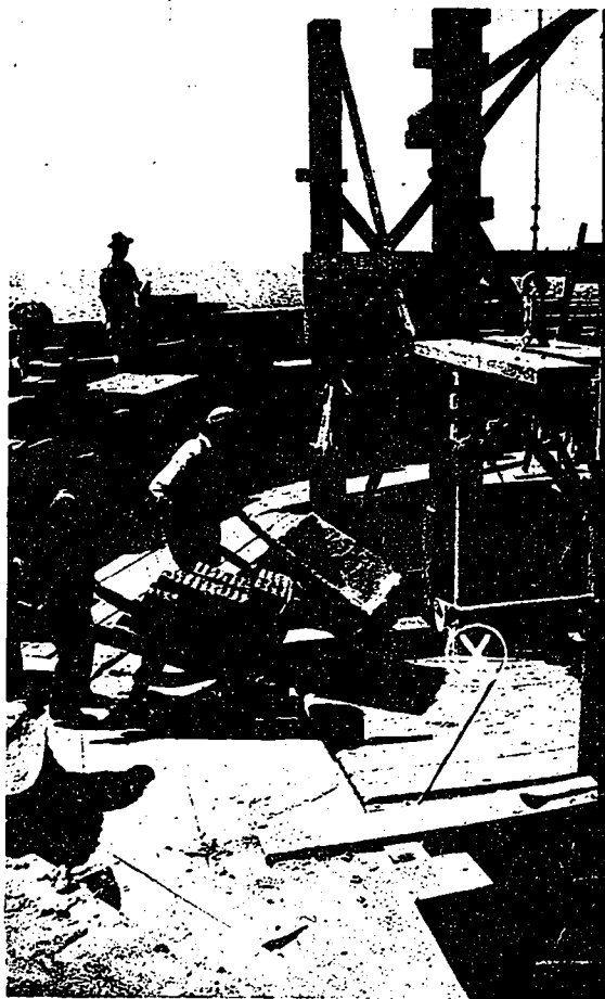
VIEW OF WORKMEN'S SCAFFOLD INSIDE OF STACK. THE SPEAKING TUBE SHOWN AT X IS PART OF A COMPLETE SYSTEM OF COMMUNICATION WHICH CONNECTED WITH EACH ELEVATOR.
