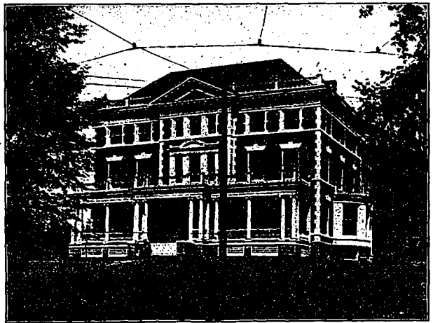
ONE OF THE MANY FINE HOMES IN WHICH THE KELSEY WARM AIR GENERATOR HAS SUCCESSFULLY SOLVED THE PROBLEM OF HEATING AND VENTILATION.
