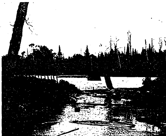
PLANT OF WOOD PRODUCTS COMPANY—VIEW OF DAM IN PROCESS OF CONSTRUCTION, SHOWING WASTE-WAY FOR THE NORMAL FALL OF THE BURNT RIVER, IN THE RECENT DRY SEASON. E. D. PITT, DESIGNING AND CONSTRUCTING ENGINEER.
