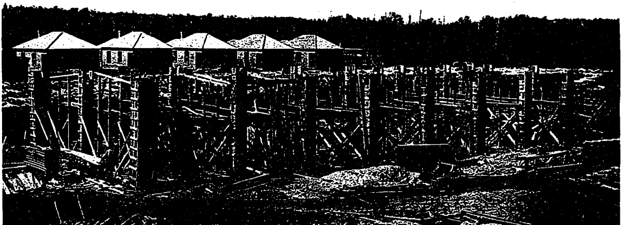
PLANT OF WOOD PRODUCTS COMPANY—FORM WORK PARTIALLY ERECTED AND COMPLETED FOR THE FIRST TOWER OF THE CHARCOAL HOUSE. THIS FORM WORK WAS PRACTICALLY ERECTED COMPLETE IN A DAY AND A HALF. E. D. PITT, DESIGNING AND CONSTRUCTING ENGINEER.
