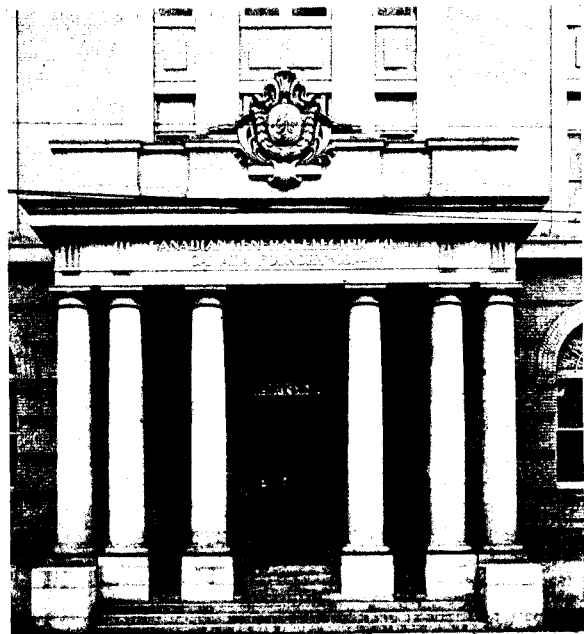
Main Entrance, Canadian General Electric Co.'s Building, Toronto. Darling & Pearson, Architects. FRED HOLMES & SONS, Contractors.
