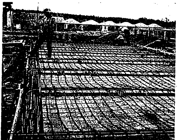
PLANT OF WOOD PRODUCTS COMPANY—VIEW SHOWING STEEL CHAIN FABRIC ON THE TANK FLOOR OF STILL HOUSE, USED IN CONNECTION WITH THE NIAGARA BAR FOR BEAMS. THIS FLOOR WAS FIGURED FOR 400 LBS. UNIFORM LIVE LOAD; IT IS NOW LOADED TO OVER 50 TONS CONCENTRATED LOAD, AND THERE IS NO APPARENT DEFLECTION AND IT IS IN PERFECT CONDITION. E. D. PITT, DESIGNING AND CONSTRUCTING ENGINEER.
