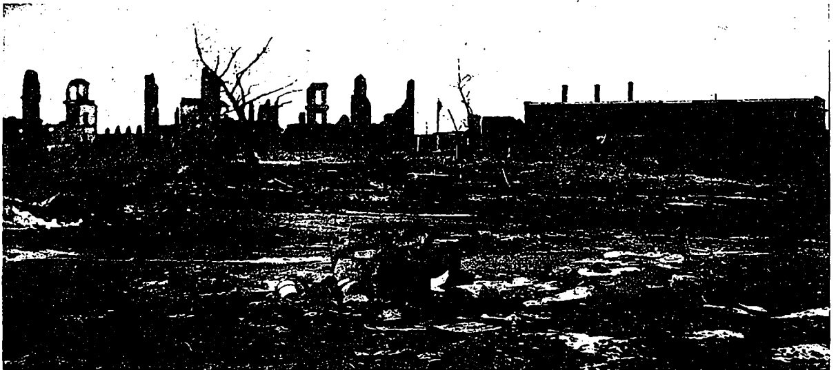
VIEW OF DISTRICT RECENTLY SWEEP BY FIRE AT PEMBROKE, ONT., SHOWING THE CONCRETE BLOCK CARRIAGE AND WAGON FACTORY OF ALEXANDER BARR WHICH WAS THE ONLY BUILDING THAT SUCCESSFULLY STOOD THE ONSLAUGHT OF THE FLAMES.
