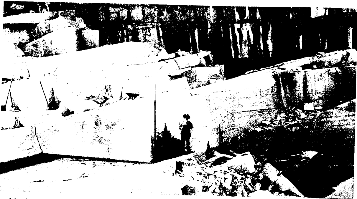
Section of Granite Quarries at Stanstead, P.Q., Showing Depth of Seams From Which Were Taken the Granite for the Column Drums and Plinth Blocks, of the Bank of Commerce, Montreal.
