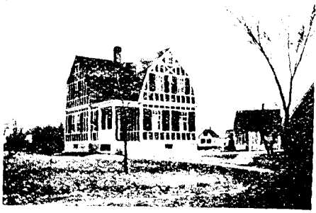
One of a group of cottages covered roof sides with our roofing.
