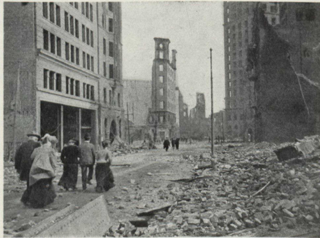
"EXAMINER" BUILDING IN CENTRE; "CHRONICLE" BUILDING TO LEFT; "CALL" BUILDING TO RIGHT
