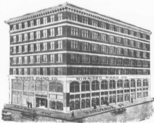
The Builder's Exchange Building, Winnipeg, just purchased by Winnipeg Piano Co., Limited.
