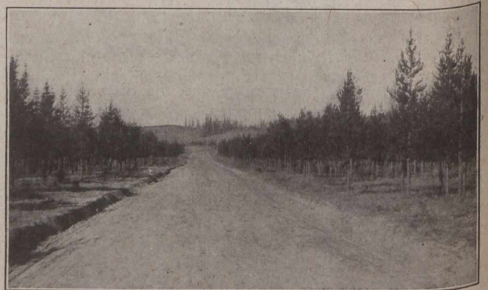
Section of Motor Road between Banff and Lake Louise, Alta. This road when completed will be 38 miles long with a maximum grade of 6 per cent. Twenty-seven miles have already been constructed.
