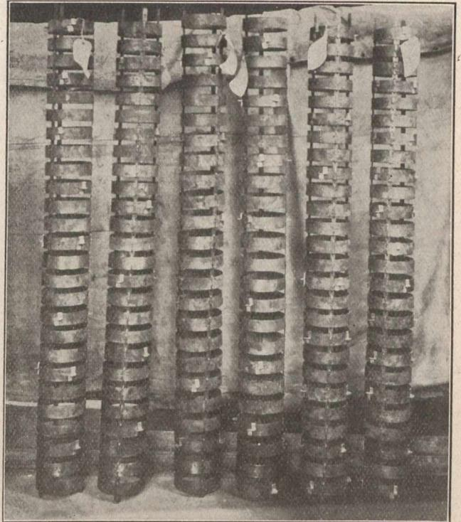
Fig. 5.—Hooped reinforcement ready to place in forms.
