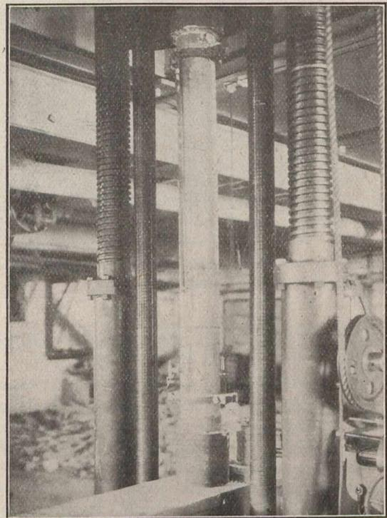
Fig. 4.—Column with longitudinal reinforcement under test.
