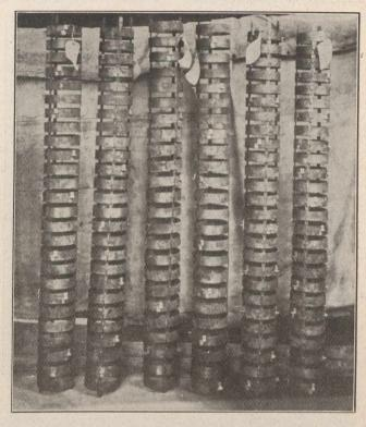
Fig. 5.—Hooped reinforcement ready to place in forms.
