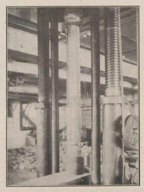
Fig. 4.—Column with longitudinal reinforcement under test.
