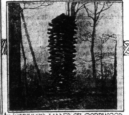
AN IMPROVED LADDER OF CORDWOOD
