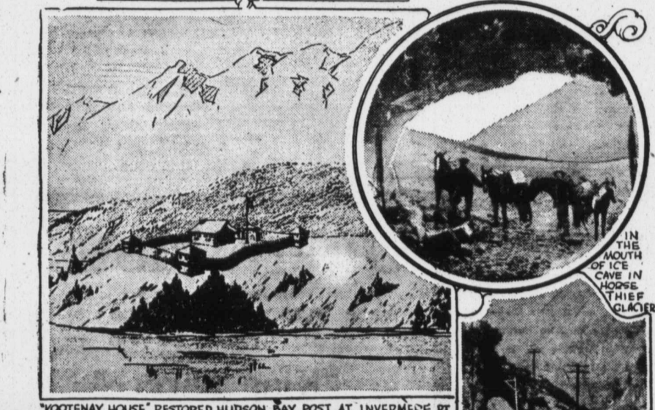
"KOOTENAY HOUSE," RESTORED HUDSON BAY POST AT INVERMERE PT. ON LAKE WINDERMERE, B. C.
