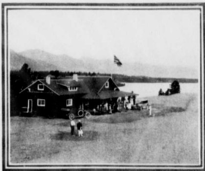
Community House, Lake Windermere Bungalow Camp
