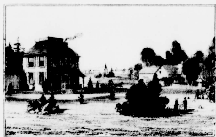
IMPROVED HOUSE FINISHED
