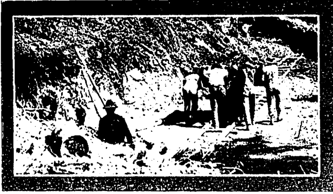
CONSTRUCTION GANG AT WORK
