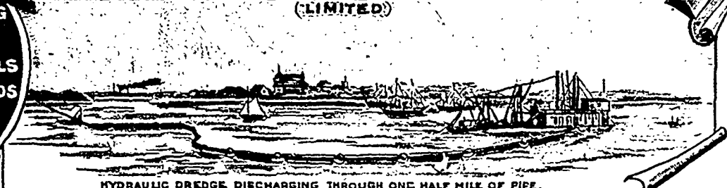
HYDRAULIC DREDGE DISCHARGING THROUGH ONE HALF MILE OF PIPE.
