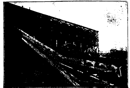
Freight and Package Elevator
