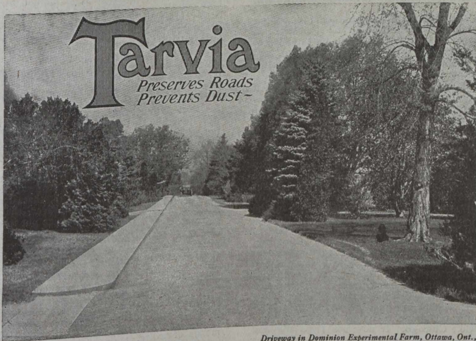
Driveway in Dominion Experimental Farm, Ottawa, Ont., Constructed with "Tarvia-X" in 1914
