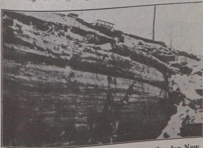
Ice-moulded Face of Escarpment, Excavation for New Customs Building, Sussex Street, Ottawa
