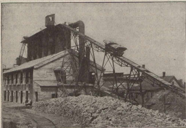
View of Complete Plant, Showing Lime en route to Kiln.
