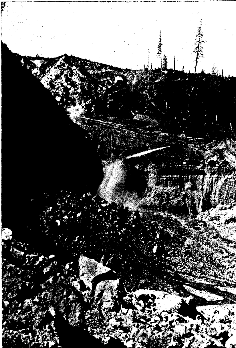
Giant on bank in Dancing Bill Gulch. Stream at work making a cut for Pipe Line.
