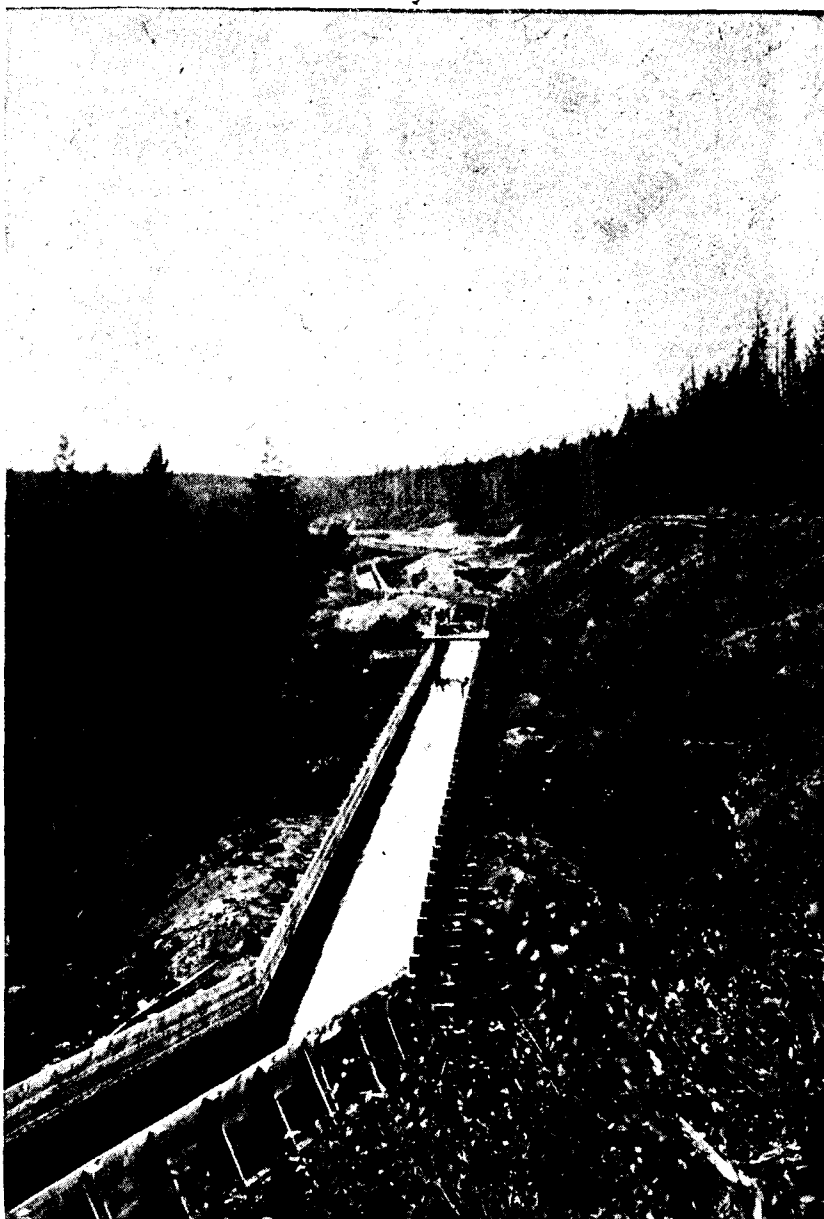
Flume on Morehead Canal, replacing Ditch destroyed by slides. See portion of destroyed Ditch on the right of Photograph.
