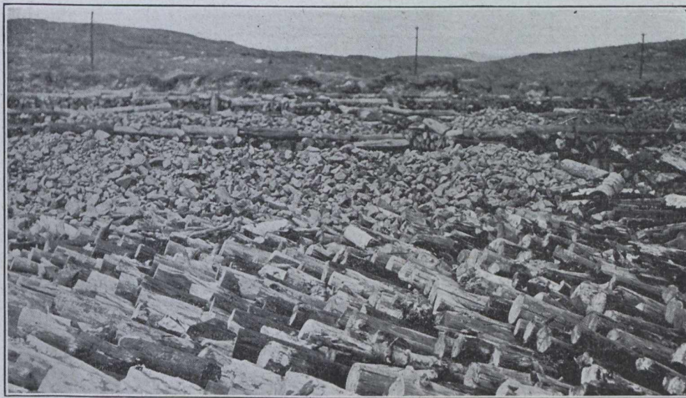
Nickel-Copper Ore on Wood for Roasting
