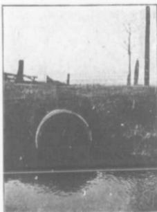
A concrete tile culvert
