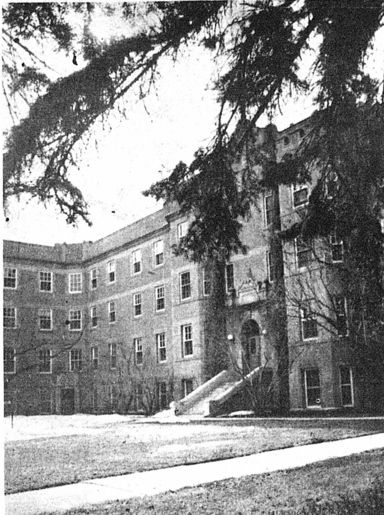
Next on the Board of Governors' list for renovations is Athabasca Hall. At a cost of about $2.16 million, the old residence will be used for office space. The entire inside of the building must be gutted and rebuilt, as well as repairs to the roof and building frame. Bill Weir
