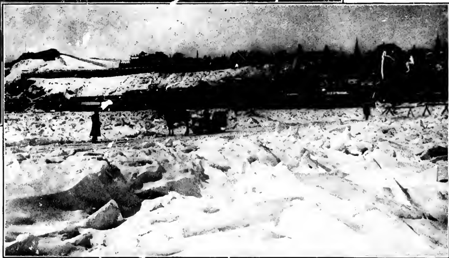
QUEBEC, SUMMER AND WINTER—THE ICE BRIDGE IN THE RIVER
