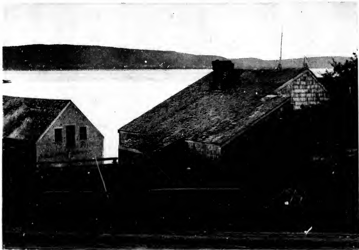
OLD HOUSE AT DIGBY
