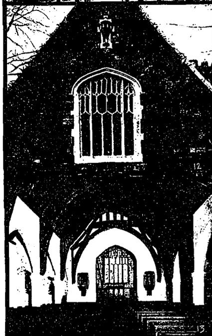
12—Gothic window and canopied niche, Second Congregational Church, Lynn, Mass., in which the under cut tracery and mouldings so necessary to the architectural success of a building of this style, is executed in concrete stone.
