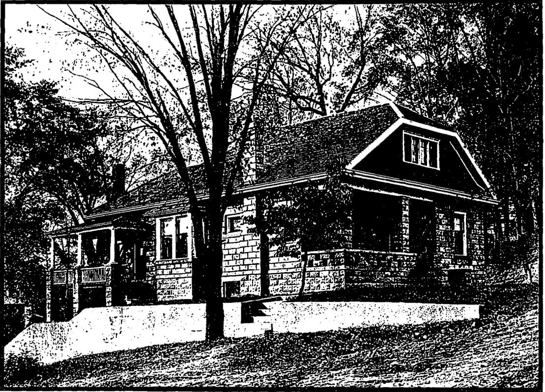
Residence of Rev. William Potter, Dundas, Ont. A Six-Room and Attic Dwelling Structure Constructed of Concrete Blocks, and Erected at a Complete Cost of \$2,600. M. H. Hewitt, Architect.
