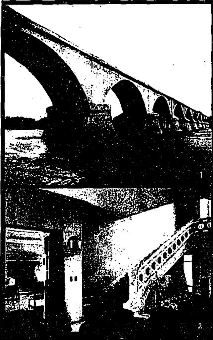
1—Huge Reinforced Concrete Bridge Built Across the Maumee River at Waterville, Ohio. This Structure is Designed to Carry Over 500 Tons on Each Span. It is 1,200 Feet Long and 45 Feet High, and Was Erected at a Cost of \$77,000. There are Twelve Spans in all, the Two Largest of which (90 Ft. Each) are Seen in the Accompanying view.
