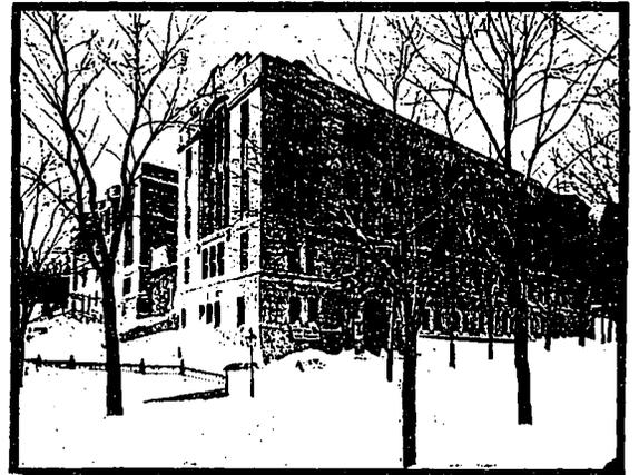
Medical Building, McGill University, Montreal. An Important Structure in Which the Interior Construction Throughout is Rendered Fire-Resisting in Character by the Use of Concrete on Galvanized Expanded Metal Lath. Brown and Vallance, Architects.
