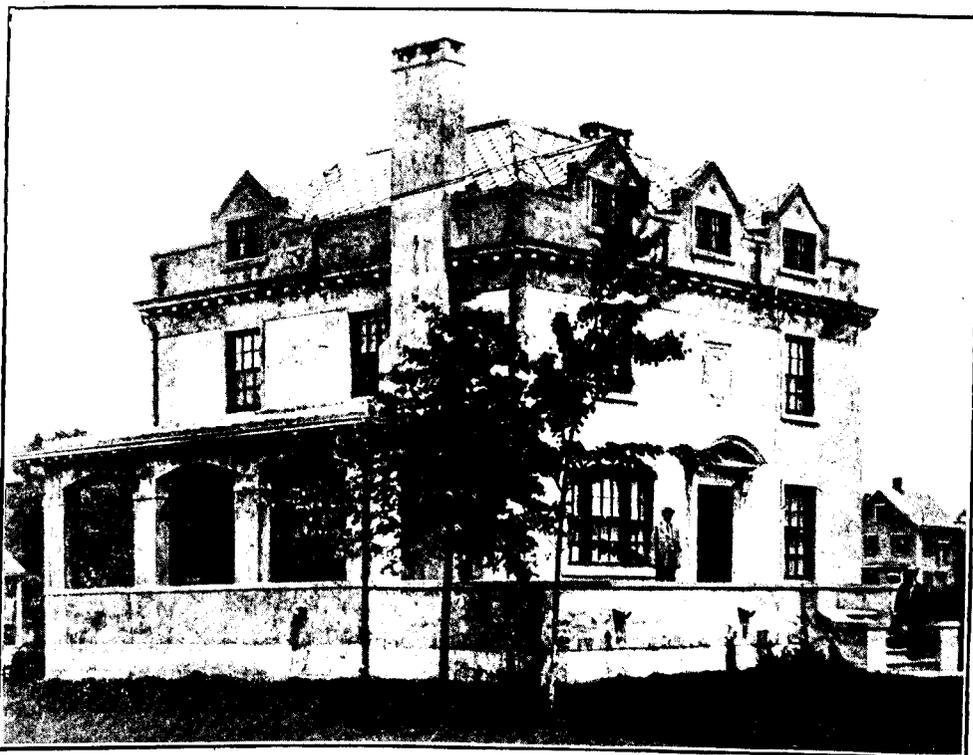
Monolithic Reinforced Concrete Residence Constructed with our System of Molds. An Absolutely Fireproof and Time-Proof Structure with Concrete Walls, Partitions, Stairs, Balustrades, Mantels, Floors and Roof. There is No Wood in the Entire House, with the Exception of the Doors and Window Frames. This House was Built at Montclair, N.J., from Plans Prepared by Mr. F. L. Ellingwood, Designer of the New Pennsylvania Station in New York, and now Head of the C.P.R. Architecture Department.
