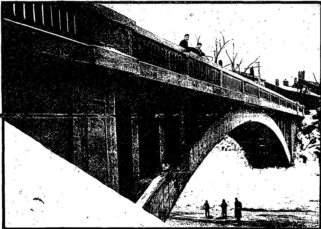
Fig. 6.—The Wadsworth Arch Bridge over the Humber River at Weston, Ont. It is Believed that the Span of this Bridge, 118 Feet 6 Inches, is the Longest Yet Attained in Concrete in Canada, and that This is the Only Completed Example of a Ribbed or Open Spandrel Arch in the Country. Barber & Young, Engineers.
