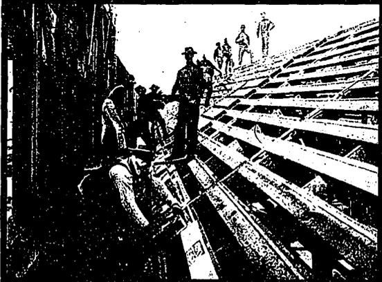
Concrete and Hollow Tile Construction. Upper View: Interior, Showing Complete Floor. Lower View: Method of Laying Tile on Concrete Roof Supports. This Type of Work Bids Fair to Attain Considerable Popularity, both Owing to Economy in Cost and the Light Yet Strong Form of Construction of Which it Admits.
