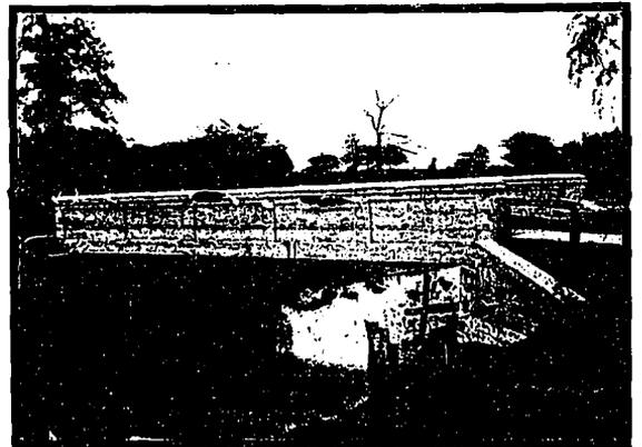
Fig. 3.—Through Girder Bridge of 50 Feet Span at Unionville, Ont. A Less Economical Type than the Deck Span of Fig. 2, but Necessitated Where the Clearance Above the Water is Restricted. Jas. McDougall, Engineer.
