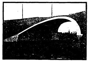
Fig. 9.—A Horse-shoe Culvert on the Toronto and York Radial Railway at Newmarket, Ont. The Close Conformity of the Lines of the Structure with the Fill Indicate an Economical Design. Barber & Young, Engineers.
