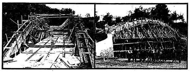
Fig 10.—Two Stages in the Construction of the Forms of the Middle Road Bridge. In this Type of Structure the Form Work Constitutes a Large Part of the Cost, but is Largely Offset by Economy of Material. Special Care was Taken to Detect and Prevent any Lateral Movement of the Trusses During Concreting. Barber & Young, Engineers.
