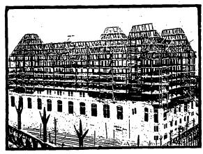
Chateau Laurier, Ottawa's Splendid New Hotel, Now Nearing Completion, and in Which the Structural Parts Throughout are Protected by a Patent Welded Fabric and Concrete Plaster Applied to Metal Lath. Ross and McFarlane, Archi-
