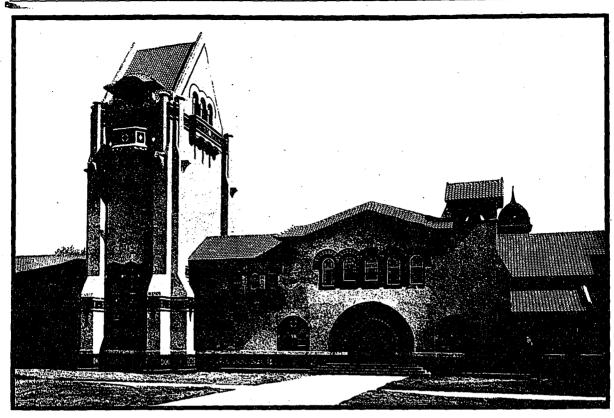
Administration Section and Tower, State Normal School, San Jose, California. A Recently Completed Monolithic Structure which is Noteworthy both as an Example Showing a Frank and Consistent Use of Concrete in Exterior Wall Treatment, and as an instance which Forcibly Demonstrates the Opportunities Concrete Affords for Architectural design in the Hands of an Architect Who Fully Appreciates the Possibilities of His Material. W. D. Coates, Jr., Architect.
