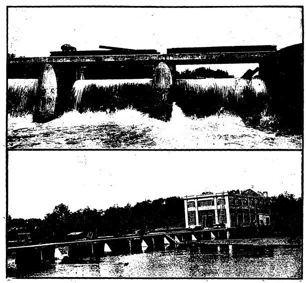
Reinforced Concrete Waterworks Dam and Power House Built for the Municipality at Peterboro', Ont. William Kernedy, Jr., Engineer. A Character of Work for Which Concrete is Particularly Adapted. Bishop Construction Company, Contractors.
