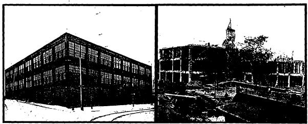
Reinforced Concrete Factory of the Peabody Manufacturing Company, Walkerville, Ont. Showing the Completed Structure and the Form Work when the Building was in Process of Erection. Bishop Construction Company, Contractors.
