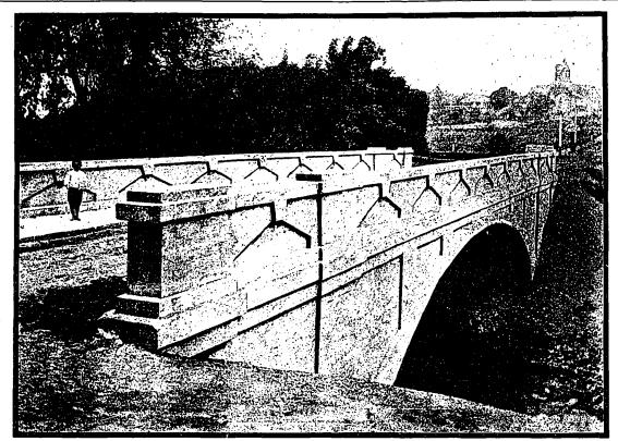
Fig. 5.—Arch Bridge of 60 Feet Span, on Timothy Street, Newmarket. This Structure Being a Permanent Bridge in a Growing Town, Special Care was Taken to Secure a Pleasing Appearance by Accentuating the Arch Ring, Relieving the Spandrels by Pilasters and Employing a Special Decorative Feature in the Railing. Barber & Young, Engineers.
