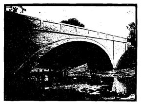
Fig. 4.—A Comparatively Plain but Pleasing Arch Bridge of 70 Feet Span at Kirkham's Mills, Township of Scarboro'. This is a Type of Permanent Structure Suited to Rural Situations where the Foundations and the Rise are Satisfactory. Barber & Young, Engineers.
