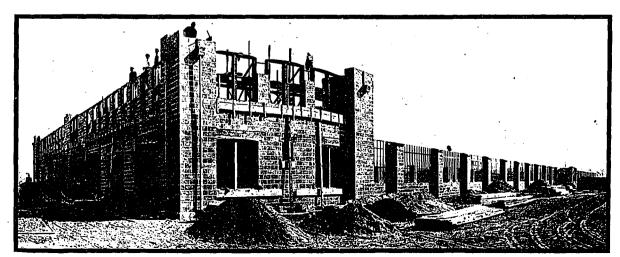
Plant of the Angidide Scale Company, Elkhart, Indiana, in Course of Construction. Showing the Cement Block Walls of a Modern Factory Before the Exterior Stucco is Applied.
