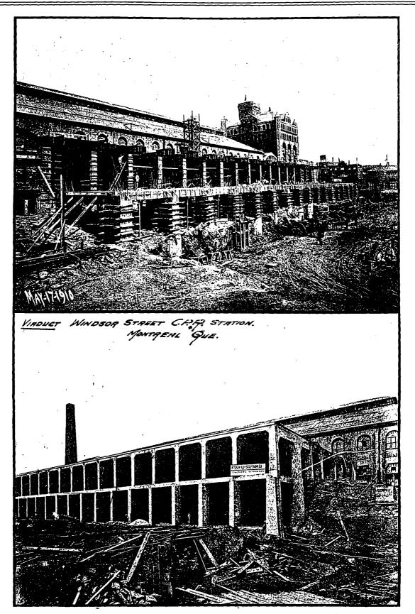
Concrete Viaduct, Windsor Street (C.P.R.) Station, Montreal. Showing Form Work, and Section of Finished Structure, Which is Designed to Carry the Heaviest Type of Locomotives and Passenger Cars. W. S. Painter, Chief Architect. Bishop Construction Company, Engineers.
