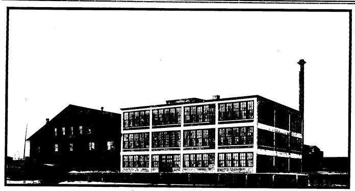
The Reinforced Concrete Factory Erected for the Ford Motor Co. of Canada, 72 feet by 88 feet. Albert Kahn, of Detroit, Architect.
