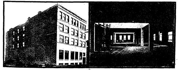
Smith Biscuit Company's Building, Vancouver, B.C. A Recent Example of the Application of Monolithic Construction to Factory Building Design. W. S. Griffiths, Architect.
