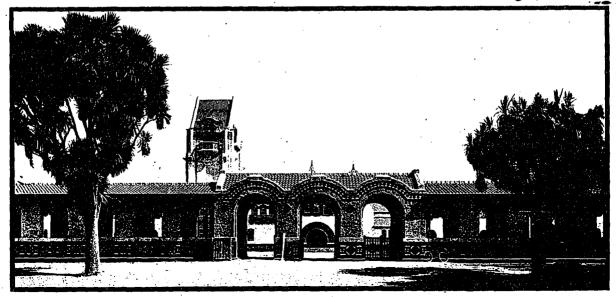
Detail of Entrance, State Normal School, San Jose, California. Showing the Red Brick and Green Tile Inlay on Grey Background, which Harmonizes Effectively with the Red Tile Roof. W. D. Coates, Jr., Architect.
