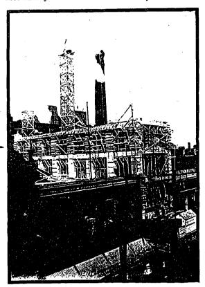
Progress View, Mason & Risch Plano Warehouse, Toronto. Showing the Form Work. The Tower on the Right Indicates the Ultimate Height of the Building. Bond & Smith, Architects.
