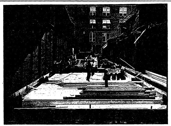
Progress View, Mason & Risch F and Warehouse. Yonge Street, Toronto. Showing the Hy-Rib Wall (partly plastered) Which was Put in Position to Enclose the McKendry Millinery Store on the South Lot Before the Brick Work of the Intervening Party Wall was Carried Up. Bond & Smith, Architects.
