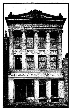
Merchants Fire Insurance Company's Building, Toronto. A Further Example Showing the Use of Manufactured Stone in Exterior Wall Treatment. Beaumont Jarvis, Architect.
