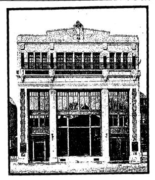
Garage of the Ontario Motor Car Company, Toronto. Showing a Richly Detailed Exterior of Cement Stone Inset with Red Brick Panels. Smith, Henchman & Grill, Architects.
