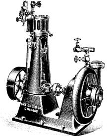
Goulds' Centrifugal Direct Connected
