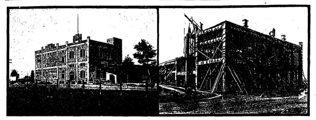
Sudbury Brewery, Sudbury, Ont. A Reinforced Concrete Building in which the Floors are Designed to Carry the Outside Brick Walls.
