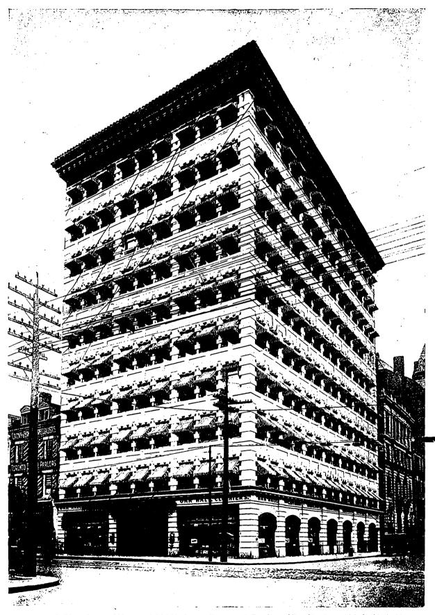
The Lumsden Building, Corner of Yonge and Adelaide Streets, Tovonto. A Ten-Story Office Structure which Strikingly Illustrates the Architectural Use of Concrete Stone in Exterior Wall Construction. It is the Largest Building in the World Entirely Faced with Manufactured Stone. J. A. Mackenzie, Architect.
