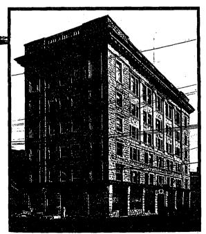
Grain Exchange, Calgary. Faced with Calgary Stone, and Possibly the Largest Reinforced Concrete Commercial Building Between Winnipeg and Vancouver. Hodgson & Bates, Architects.
