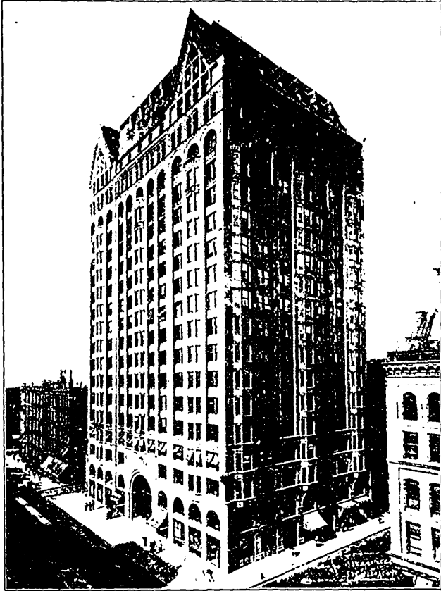
STEEL STRUCTURE, MASONIC BUILDING, CHICAGO.
